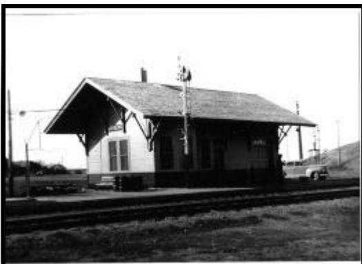
The depot after it was completely restored in Sterling
