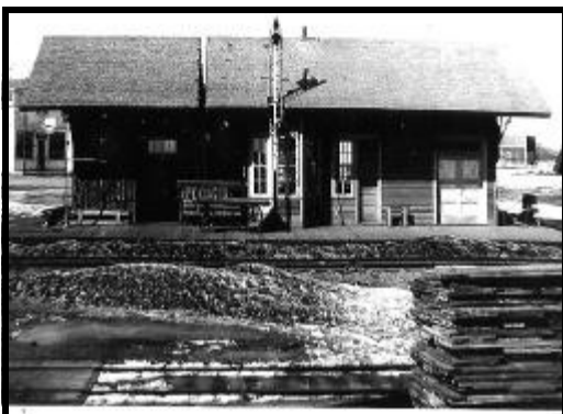
The Sterling Depot during downsizing. Note the cut in the roof!
